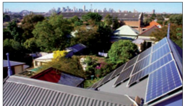
**Figure 2** BP Solar PV panels installed on the roof of the Olympic Village in Sydney, Australia. Grid-connected PV, feeds energy back into the electricity grid during the day, and is taken from the grid at night making it the most rapidly growing PV market.
