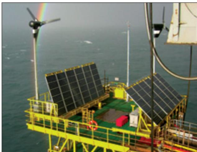
**Figure 1** A view of Shell's Cutter Platform in the Southern North Sea, installed in 2006. The wind and solar devices power the platform and are installed purely for commercial reasons (Sweeney, pers com). The installation itself was based on offshore wind farm technology.
